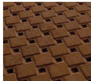
Figura 2. Pavimento adoquinado permeable. Fuente: Permeable Interlocking Concrete Pavement. A comparison guide to porous asphalt and pervious concrete.
