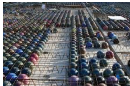
Figura 3. Sistema Bubble Deck. Fuente: www.bubbledeck.com The Sustainable Concrete guide. Strategies and Examples. Andrea J Schokker. U.S. Green Concrete Council.
