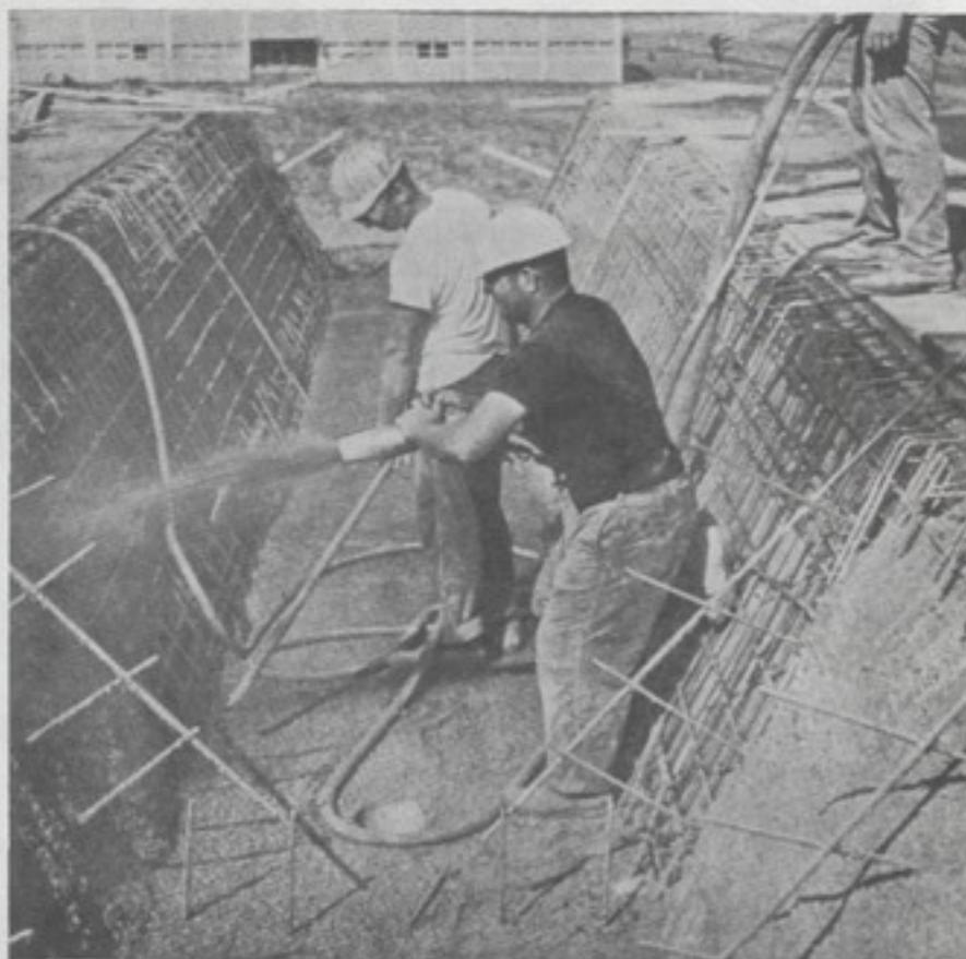
**CONCRETO INYECTADO A PRESION
